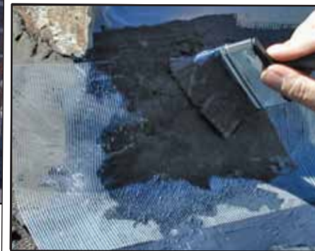
For added strength and flexibility, a fiberglass fabric is embedded between 2 coats of FlashSeal Elastomeric Sealant
